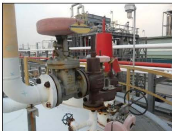
Pressure Vacuum Relief Valve
